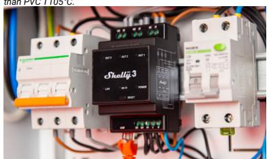
Before starting the mounting/installation of the Device, check that the breakers are turned off and there is no voltage on their terminals. This can be done with a phase tester or multimeter. When you are sure that there is no voltage, you can proceed to connecting the cables.
