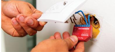
If you are using DC power supply, connect the wires as shown on **fig. 2**. Connect the load to the O terminal of the Device and the DC+ wire. Connect the GND wire to a ⊥ terminal of the Device.
